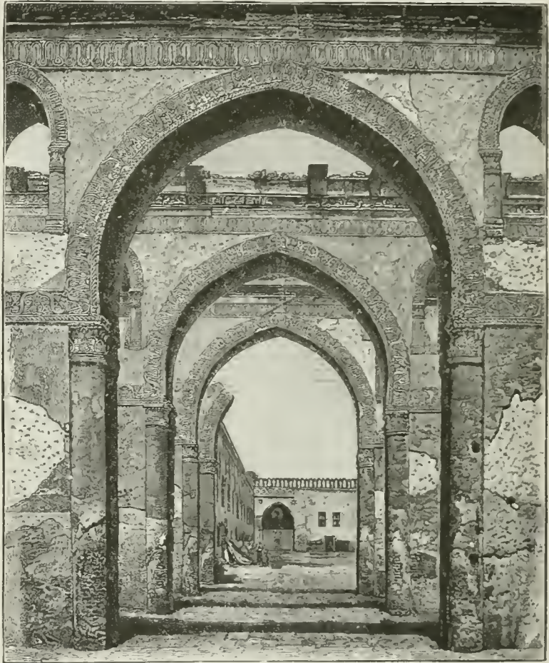
NO. 156.—ORNAMENTAL PLASTER WORK ON THE ARCADES IN THE MOSQUE OF IBN-TULUN, NINTH CENTURY.
